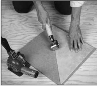
Fig. 27 - Roll the cut edge to form a slight radius.
