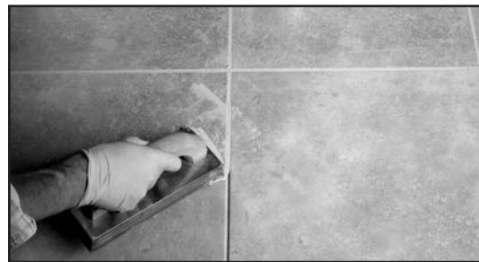
Fig. 29 - Extend grout a few inches into the next row.
