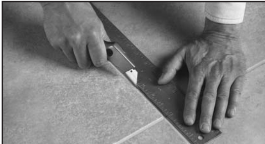
Fig. 36 - Cut along the center of the grout line after heating it.
