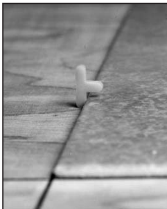
Fig. 12 - Use spacers with one leg removed.
