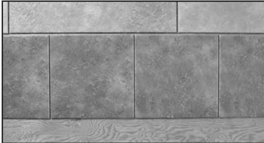
Fig. 21- An alternative to using different spacer sizes is to off-set the joints.
