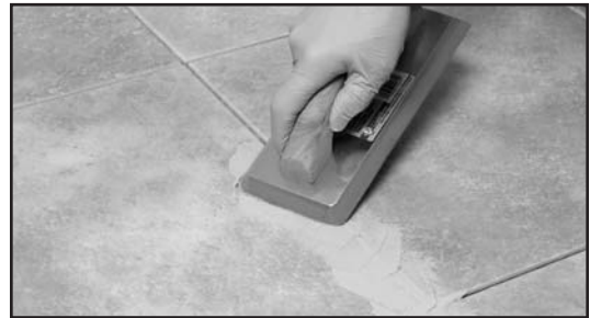
Fig. 28 - Pack the grout into the joints.
