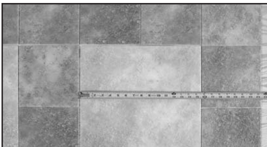
Fig. 22- Determine the dimensions for the pattern repeat.
