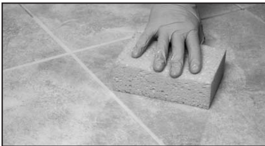
Fig. 31 - Wipe diagonally across the joints to remove excess water.
