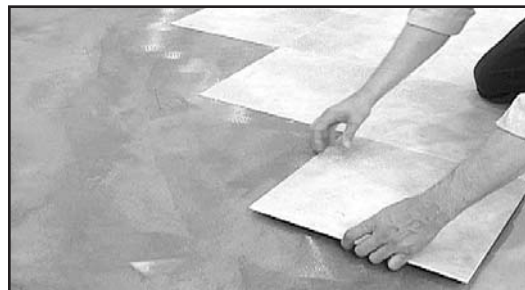
Fig. 15 - Install ungrouted floors following a stair-step pattern.
