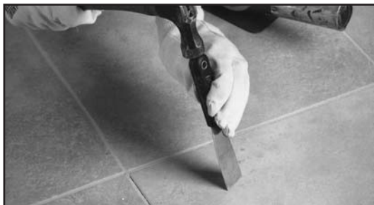
Fig. 37 - Drive a putty knife into the heated area and pry upward.
